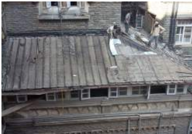
The above three images show damaged roof members at multiple locations in the building.
