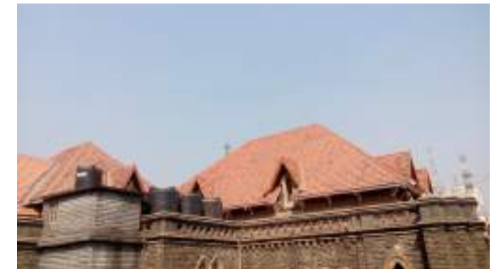
The restored roof.
