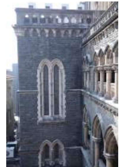
Some images of restored exterior or façades of the buildings.
