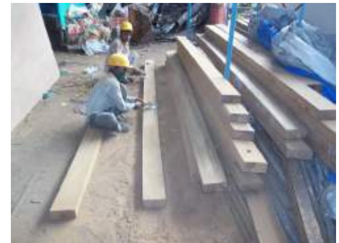
Finishing the timber rafters and stacking.
