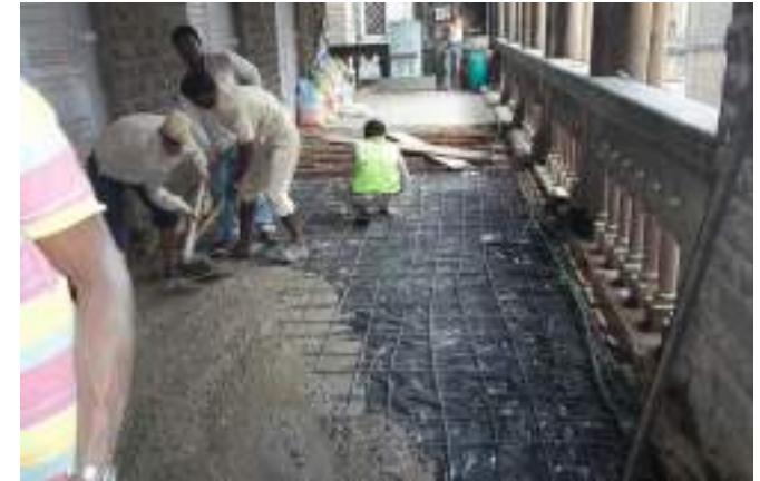
Last image below: The casting of R.C.C slab
