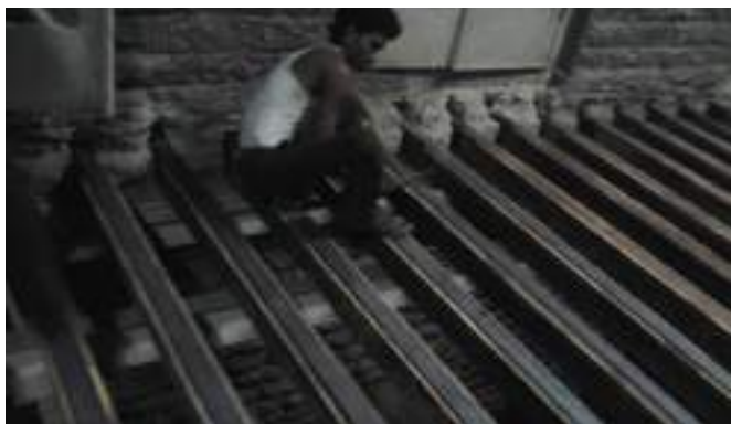
The fixing of M.S plates over the rafters.
