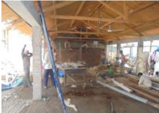
Constructing the canteen block.
