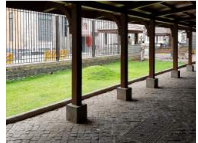
The newly made covered walkway from the High Court building to the P.W.D building. The image also shows the compound walls with grills.
