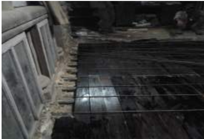
Right last: Laying of cement tiles.
