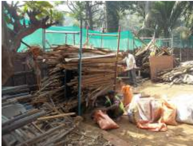
Stacking of roof tile battens.
