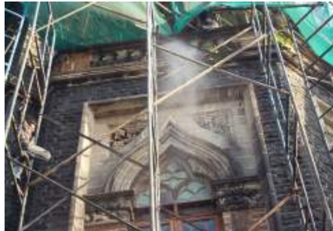
Using misting technique to remove years of dirt, dust and pollution.
