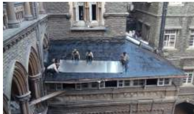
Water proofing with tar felt and G.I sheet.
