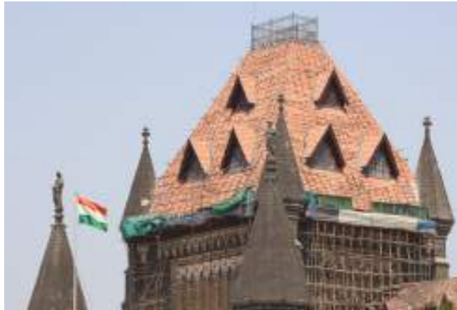
A view of the pitched roof with dormer windows.
