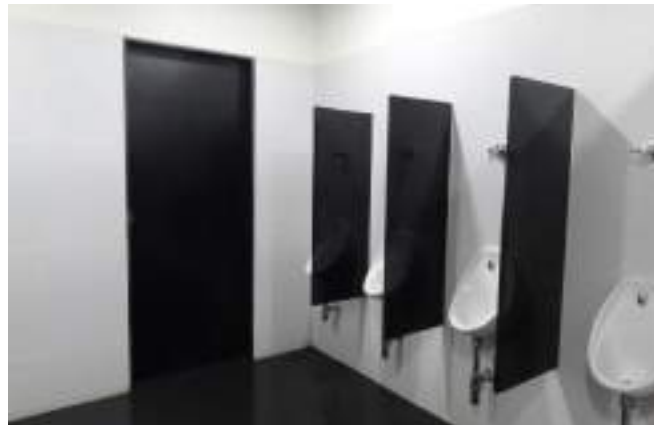
Restored public toilet.
