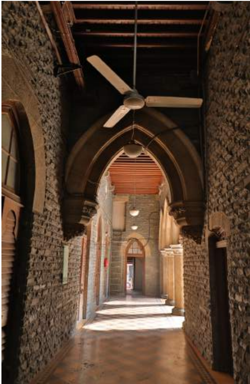
A restored corridor.
