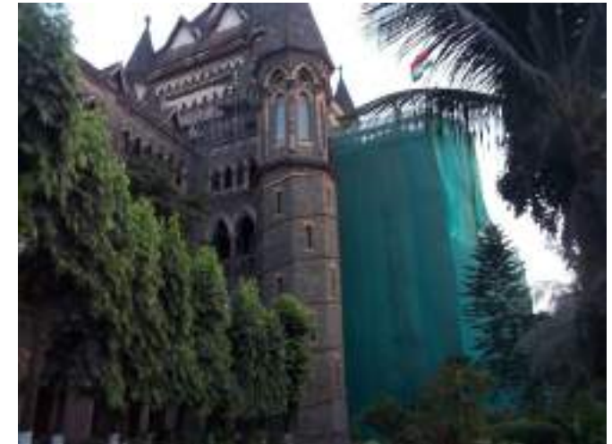
The soiled facade of the building in process of cleaning.
