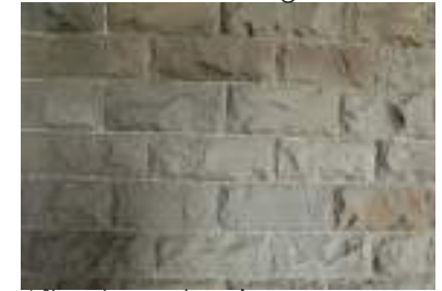
After stone cleaning.
