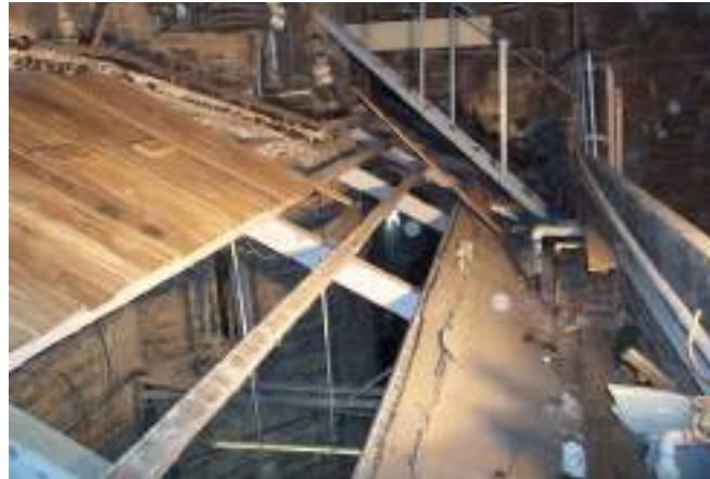
Dismantling and fixing new members for the roof.
