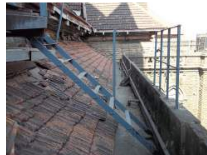
The lean to roof above the public corridors.
