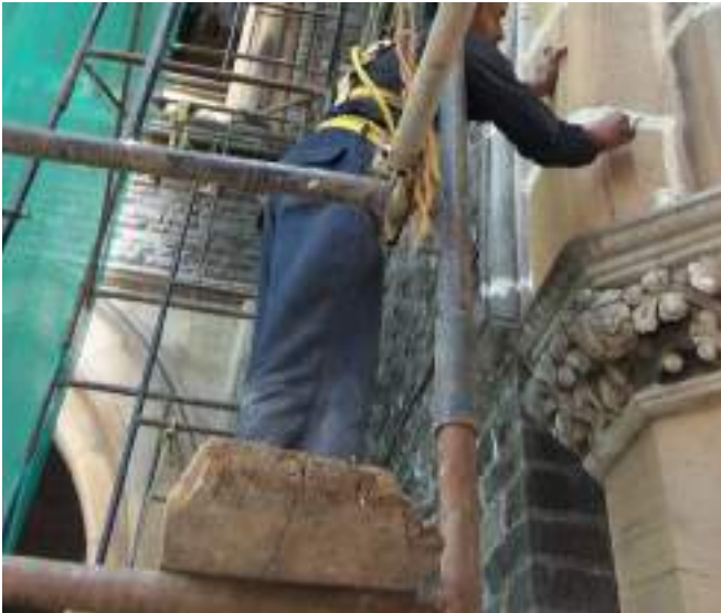
External facade restoration and pointing.
