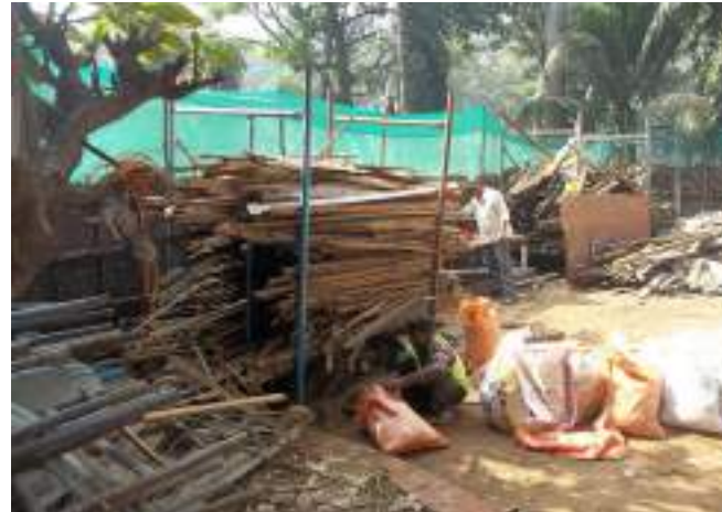
Storing and stacking of the timber sections.
