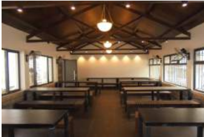
The new canteen block with benches, tables and roof.
