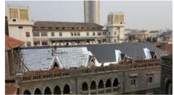
Battens fixed over the G.I sheets.
