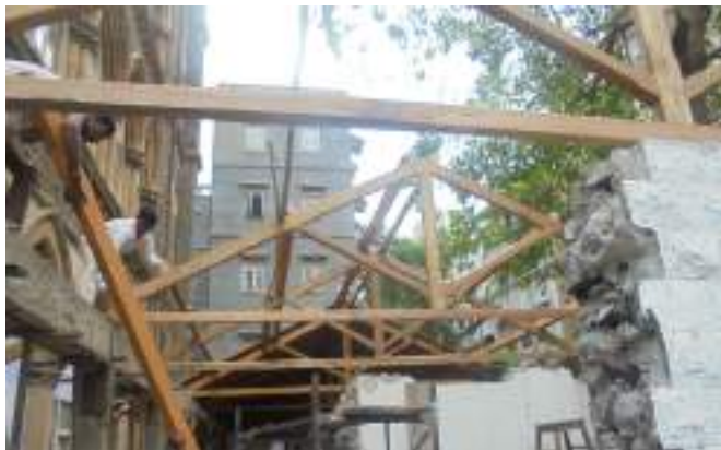
Timber roof over the new canteen building block.
