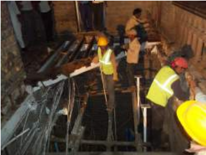
A group of workers dismantling a corridor slab.
