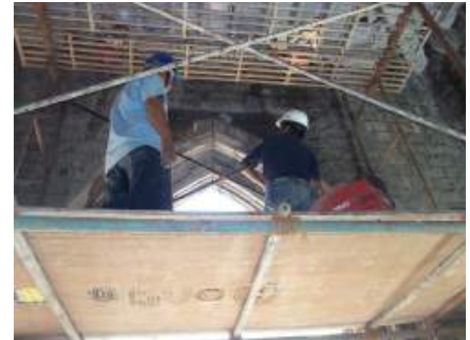
Images showing restoring the stone facade with Helifix.
