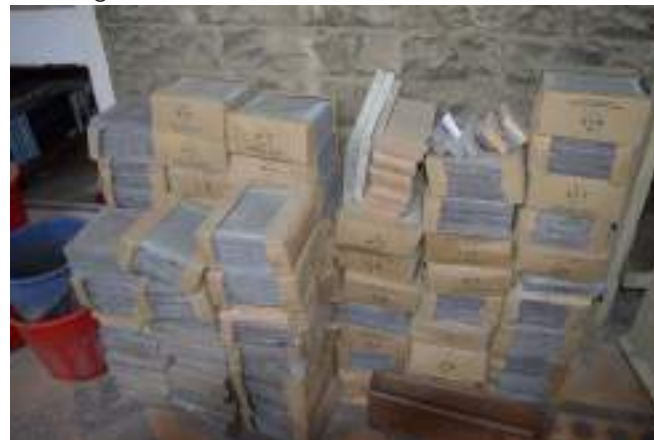
Stacking of new cement tiles on site.
