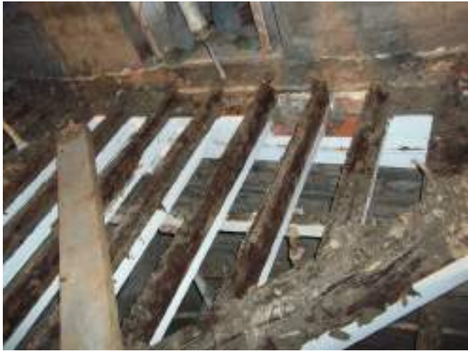
The dismantling of the slab.
