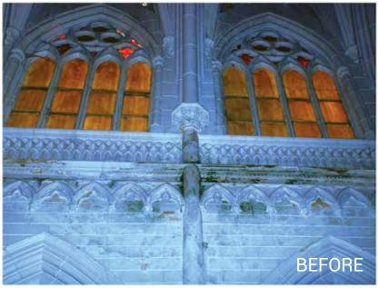
The water seepage over the years can cause patchy moss growth, especially to the members facing the exterior. The treforium level here can be spotted with a green patch which was cleared and treated later on.
