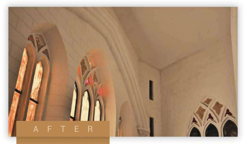
The problem of dampness and flaking was grave throughout the church building. The corners were especially damp and wet. Hence it became very important to treat the leakage to stop seepage further. All the windows in the church were made water tight.
