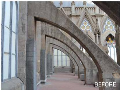
The flying buttresses are an important structural element of the church. The upper portion is arched which transfers the load below. The previous interventions were done in cement where the threat of further deterioration was possible.
