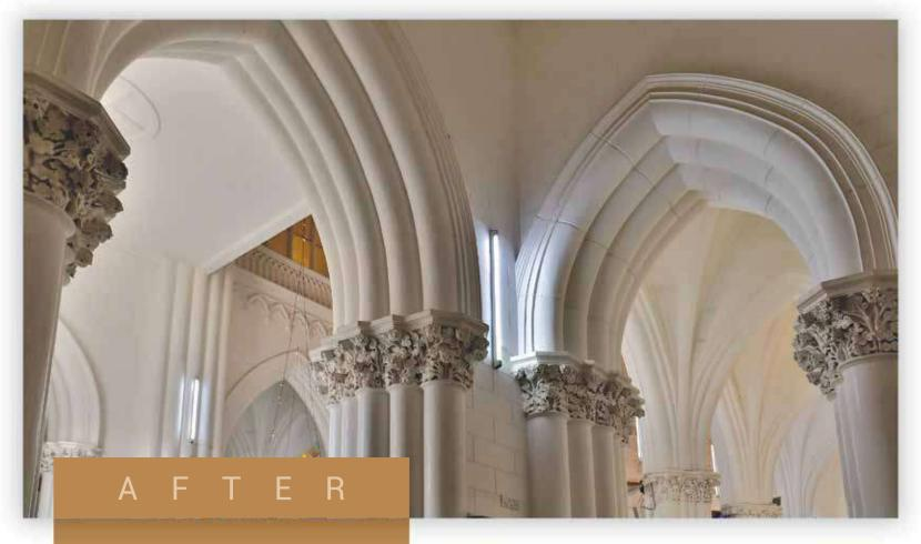
The series of arcades supported on piers in the interior of the church along the isles needed repairs, which received lime and was followed by lime plaster. The arcade did not show major signs of dampness but was in a dire need of a facelift. Some of the crockets showed signs of cracks and few were in a broken state. The fine moldings were restored back skillfully using lime.
